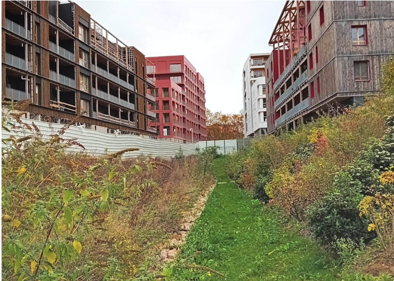
Separation wall within the Ecoquartier under construction
