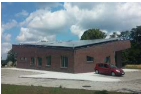
Health Centre in Gierałtowiec Municipality (Przyszwice) with 126PV on the roof [1].
