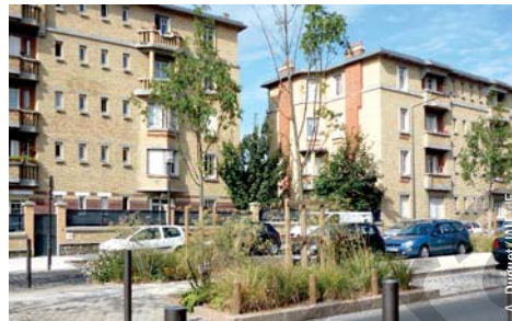
Stains: the main road has been refurbished, integrating parking spaces and a new and more up-to-date planting.
