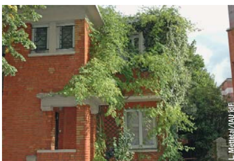
At Champigny, nature regains its freedom with climbing plants decorating the front of the buildings that face onto public spaces.
