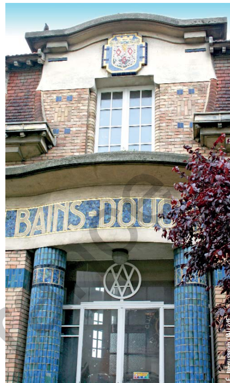
Among the numerous facilities of the garden city of Orgemont at Argenteuil, only public baths are closed, looking forward to another use.
