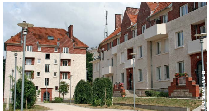
At Champigny-sur-Marne, the apartment blocks form a U-shape around a courtyard, now with restricted access.
