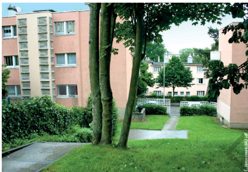
The garden city of La Butte-Rouge at Châtenay-Malabry.
