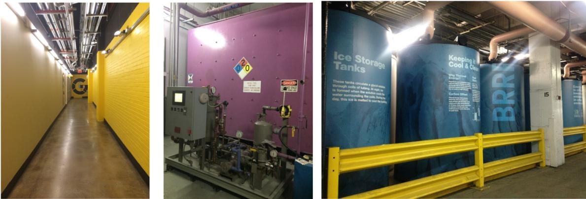
Figure 25. Interior of 111 Eighth Avenue. With fuel tank and thermal storage. Credit =©Cécile Diguët and Fanny Lopez, 2018.
