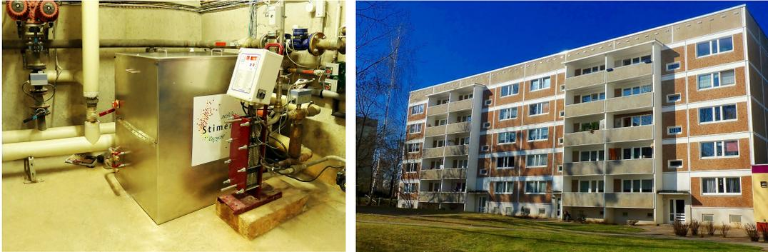
Figure 27. Stimergy digital boiler installed in a building in Échirolles with the OPAC 38, Stimergy. Credit =© Stimergy, 2018.
