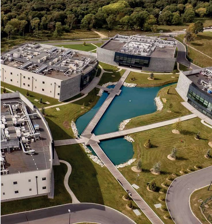
Datacenter, Paris-Saclay © Data4
