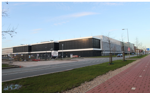
The Schiphol-Rijk sector in the municipality of Haarlemmermeer has a large number of data centers, like this Digital Realty (Interxion) one.
