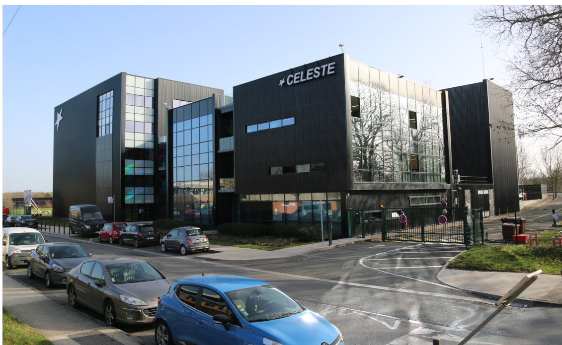
Data center « Marilyn » de Céleste, located in the Cité Descartes in Champs-sur-Marne. Source : L'Institut Paris Region, 2021.
