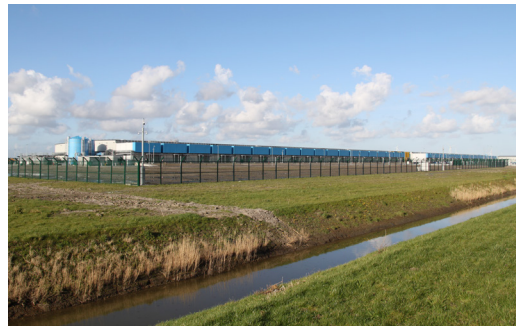
In Hollands Kroon, north of the province of North Holland, hyperscale data centers are installed, like this Google one. Several other Microsoft data centers are located nearby.
