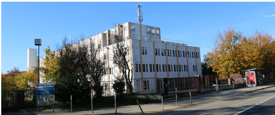
Among the data centers in the Paris region, former telecom buildings as in Vélizy-Villacoublay (above), new constructions as in Marcoussis (p. 17 top) and transformed office buildings as in Lognes (p. 17 bottom, now closed).
