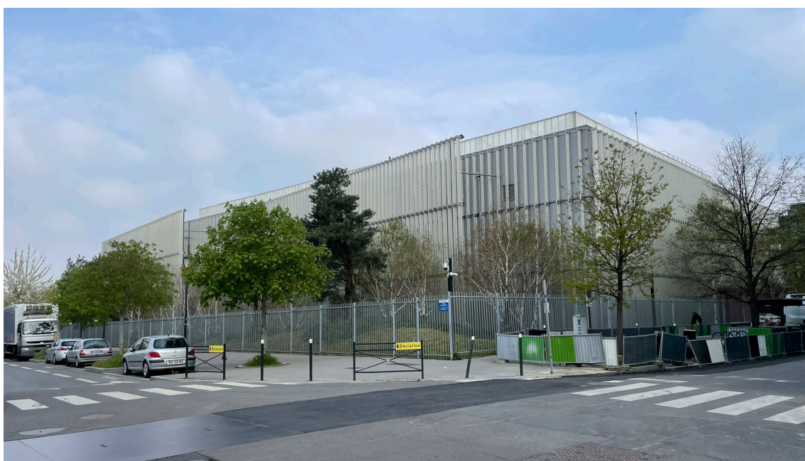
Two data centers installed in the Plaine Saint Denis: Equinix's PA6 in Aubervilliers, built in 2008, (left) and Digital Realty's (Interxion) PAR5 in Saint-Denis, built in 2009 (right). Source : L'Institut Paris Region, 2023
