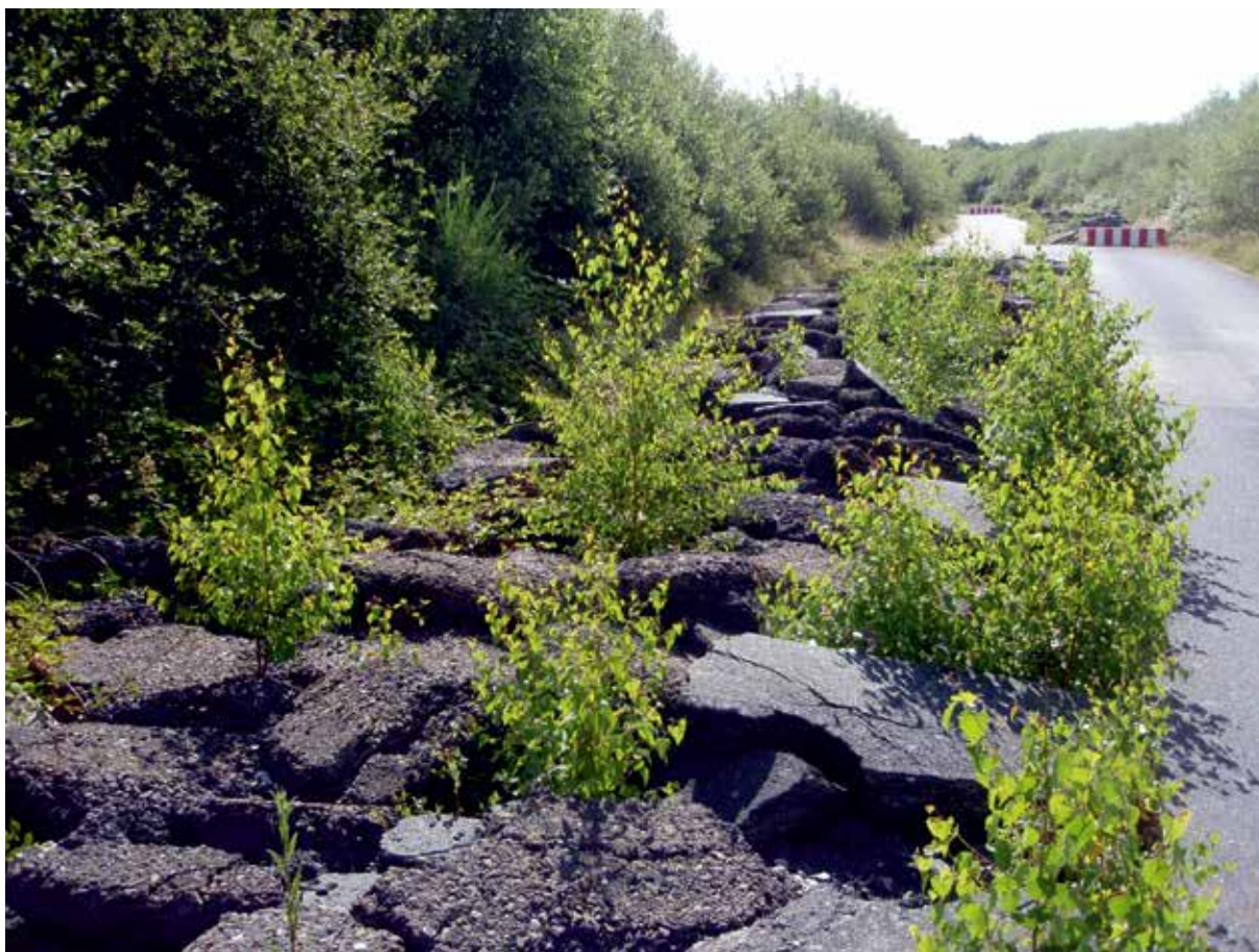
Crushed asphalt gives way to spontaneous vegetation on an old road in Saint Jacques de la Lande. © Yann Laurent
