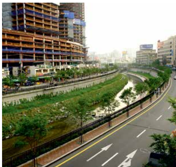
The Cheonggyecheon restoration project was centred on revitalising the Cheonggyecheon Stream that had been covered for decades by a highway overpass ©Global Designing Cities Initiative
