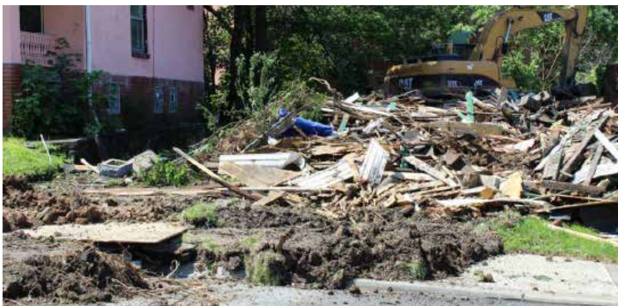
Demolition in Cleveland. ©Turo and Gardiner, 2020 [23]
