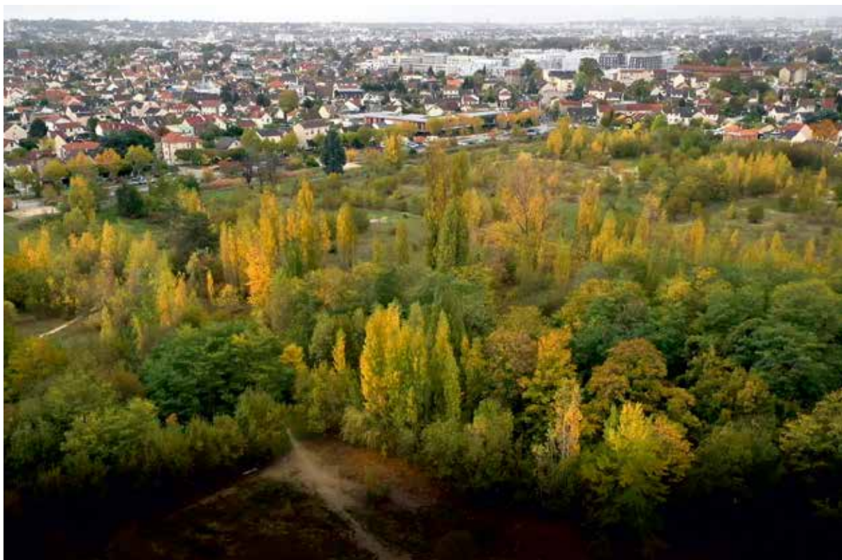
The former Kodak industrial brownfield was demolished and replaced by a park with a wide variety of habitats ©CDC Biodiversité
