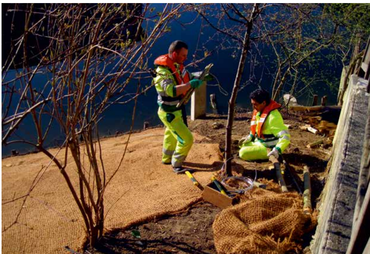
Willow spiling by Association Espaces on the Île Saint-Germain at Issy-les- Moulineaux to stabilise and replant the riverbank. ©Association Espaces
