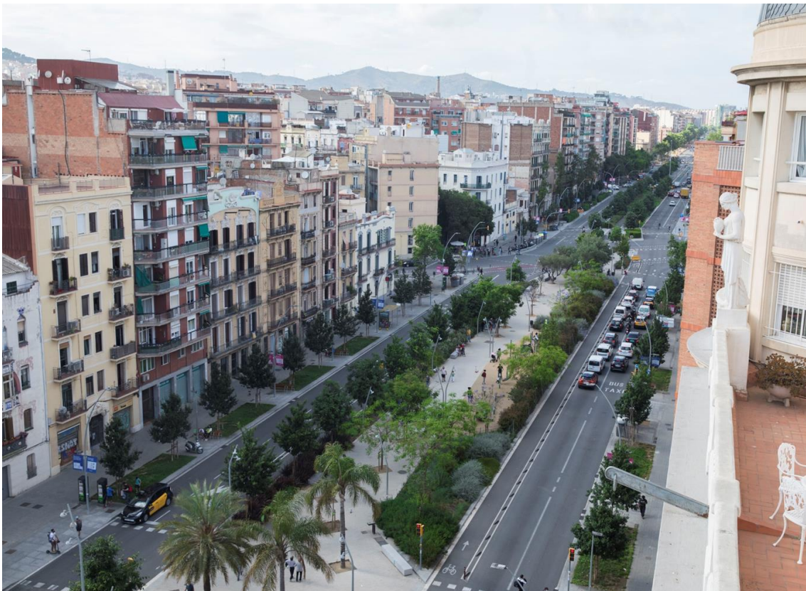
The Meridiana at the same place in 2019 as green and civic axis with only two lanes for car traffic, two bus & taxi lanes, two bicycle lanes, large planted sidewalks and a wide central green rambla. Traffic has been reduced dramatically since the late 1990s and the social use of space has increased sharply. Only 23% of space is now devoted to vehicular traffic and 67% is for the people, fauna, flora, soil and water. This kind of street greening may help Barcelona to mitigate the summer climate heat in the future. © Ajuntament de Barcelona
