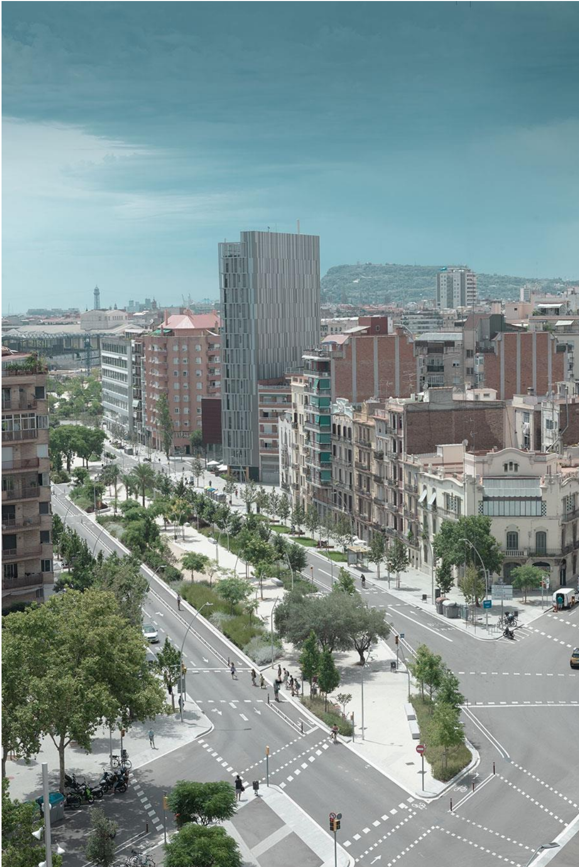
The Meridiana project is a flagship of the Metropolitan Avenues' strategy. It is remarkable in terms of public participation, design and delivery. Current traffic volumes and traffic plans of the 1970s however still strongly influence the distribution of space. Here, the shape of curbs is determined by the heavy traffic flows towards the one-way Arago street.
