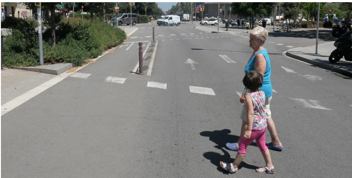
The redesigned southern section of the Meridiana in 2022. New pedestrian crossings follow pedestrian desire lines © P. Lecroart / L'Institut Paris Region
