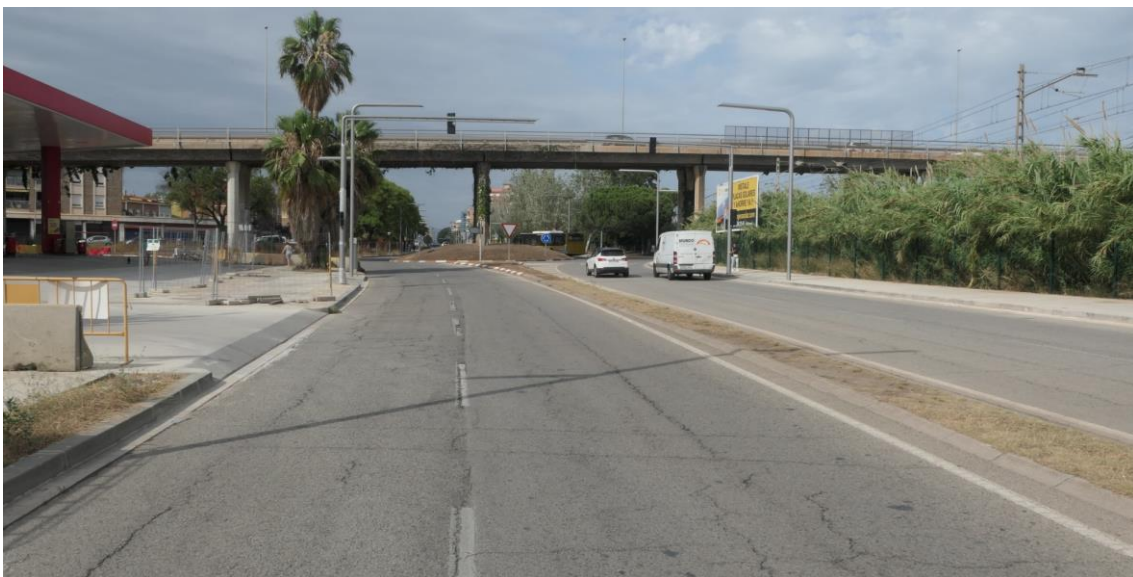
The C-245 Road as a dual carriageway in the municipality of Gavà © P. Lacroart / L'Institut Paris Region
