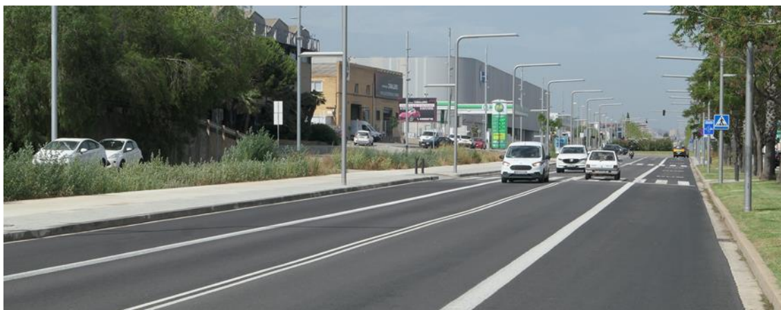
The new C-245 with widened sidewalks, 2+1 bus lanes and 2+1 lanes for general traffic © P. Lacroart / L'Institut Paris Region
