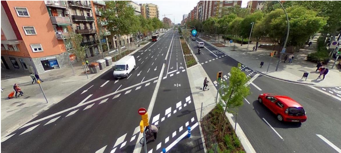
Meridiana after , Section 2. The planted median bikeway narrows to the north as the road supports heavier traffic © Ajuntament de Barcelona
