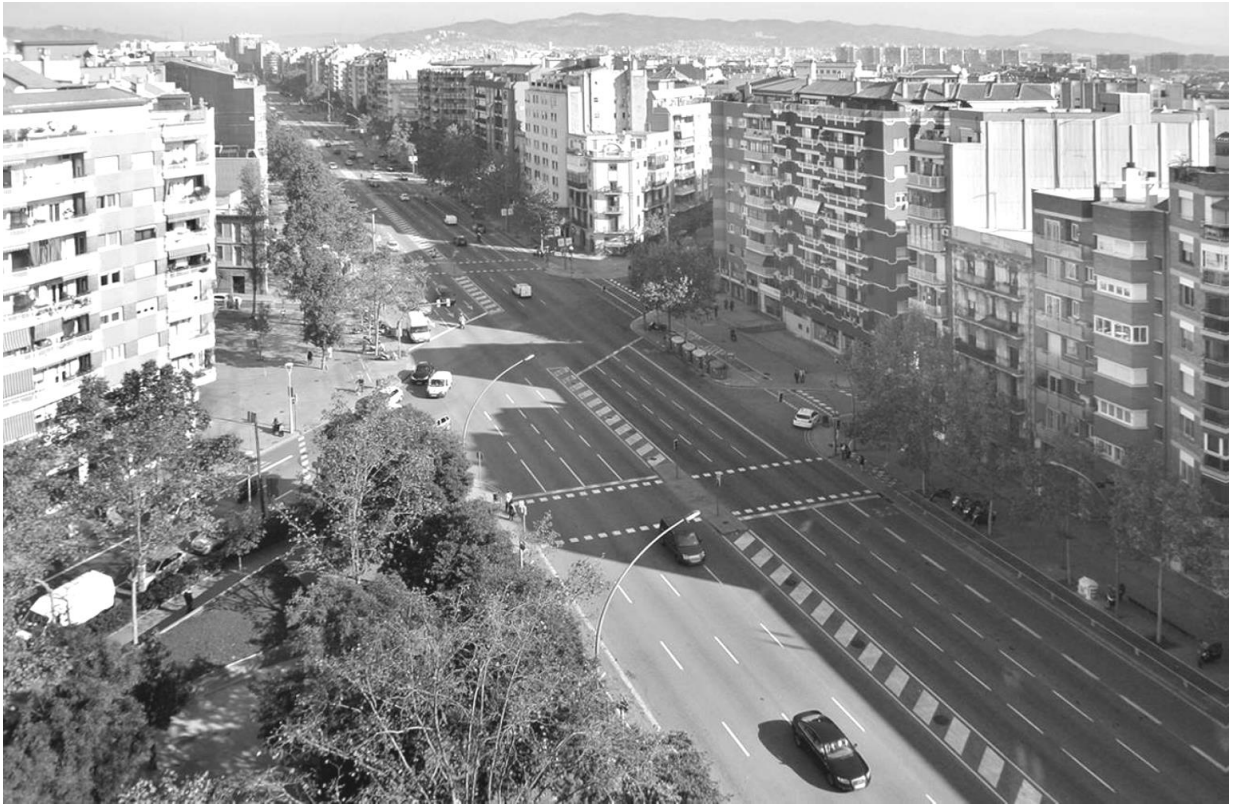
The 8-lane wide avinguda Meridiana at carrer de Mallorca before transformation © Ajuntament de Barcelona
