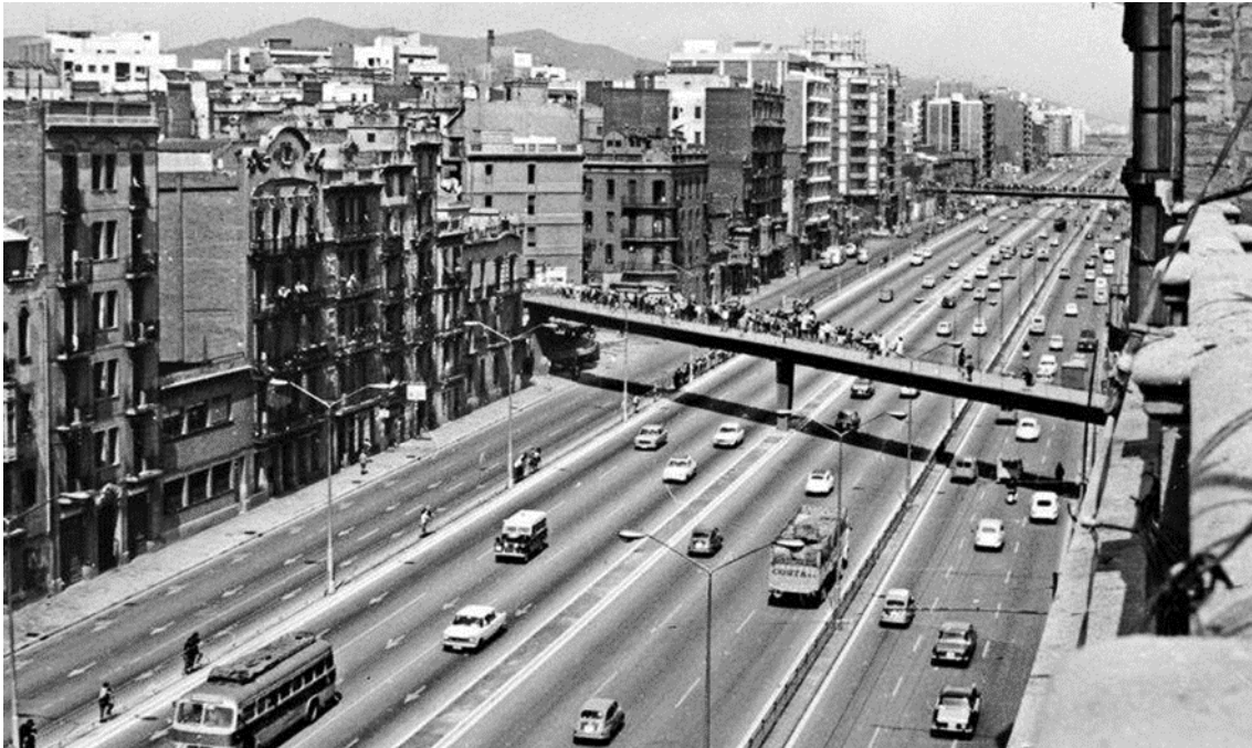
The Meridiana at Arago street transformed into a 12-lane expressway in 1965 with no trees, very narrow sidewalks and little groundfloor activity (view looking north). Almost 90 % of space is devoted to vehicular traffic. Note the pedestrians standing on separators and on the footbridges © DR
