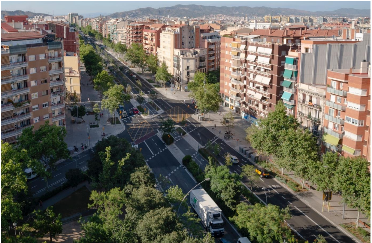
The Meridiana at carrer de Mallorca after transformation in 2022 with a large planted central median, a central 2-way bike lane, 2+2 lanes for vehicles, 2+1 lanes for busses and larger sidewalks with plant beds © Ajuntament de Barcelona
