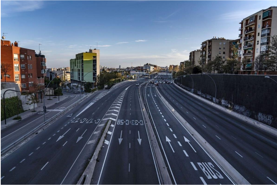
The entrance of Barcelona on the Meridiana avenue north of Ring Road (Ronda de Dalt) looking south. Notice the sheer size of the roadway (11 lanes in total here), including the bus & high occupancy vehicle lanes (HOV/VAO) coming from the C-58 expressway.
