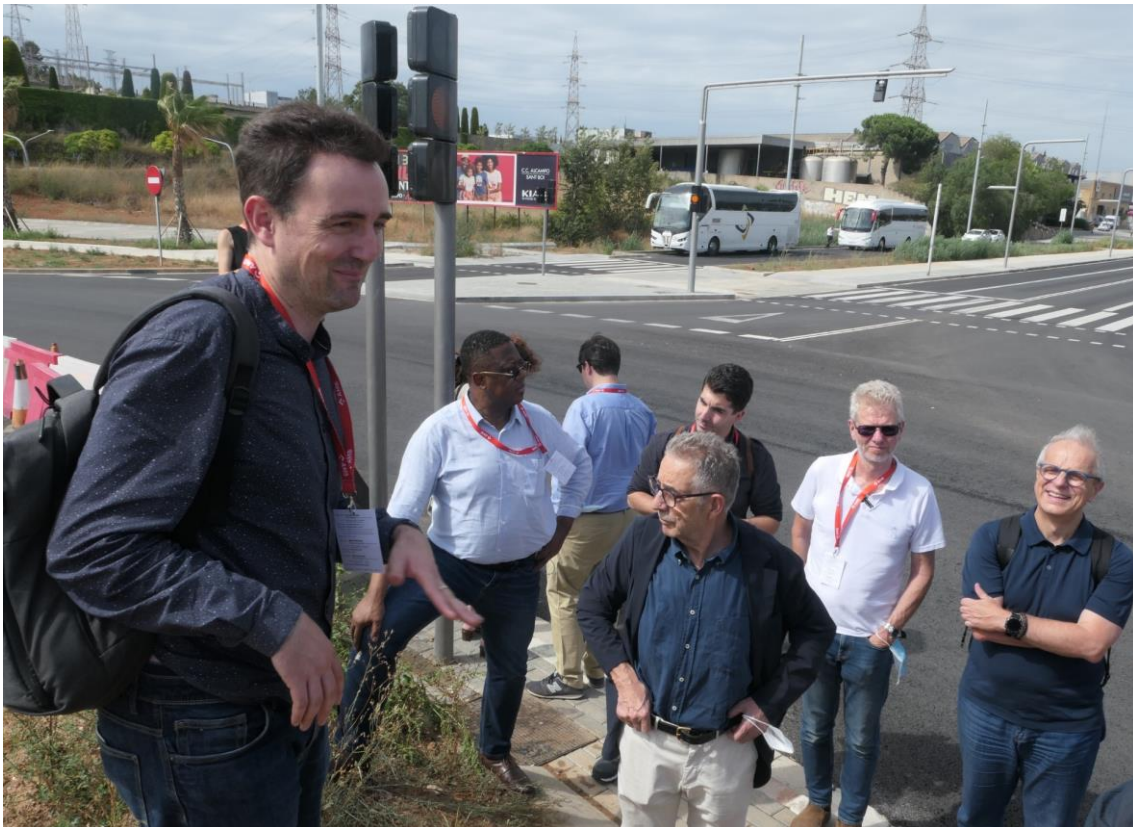
A site visit of the works on C-245 road with Joan Caba Roset (AMB) and Bernardo de Sola, lead architect in July 2022 © P. Lecroart / L'Institut Paris Region
