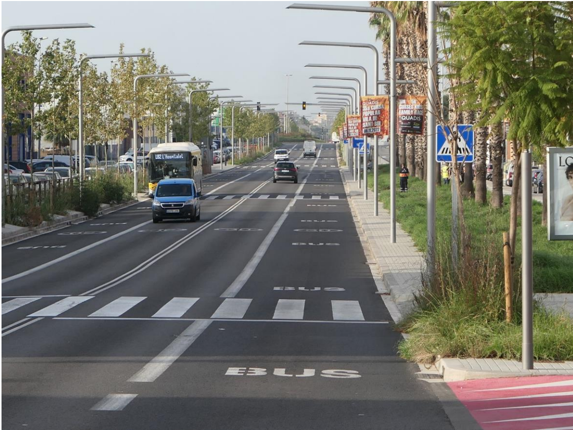
The C-245 in 2022 after delivery of the new design in Sant Boi de Llobregat with two central lanes for general traffic and two bus lanes with planted separators on both sides. Notice the narrow lanes (2.80 m for general traffic and 3.20 m for the busses) and the new lighting features.
