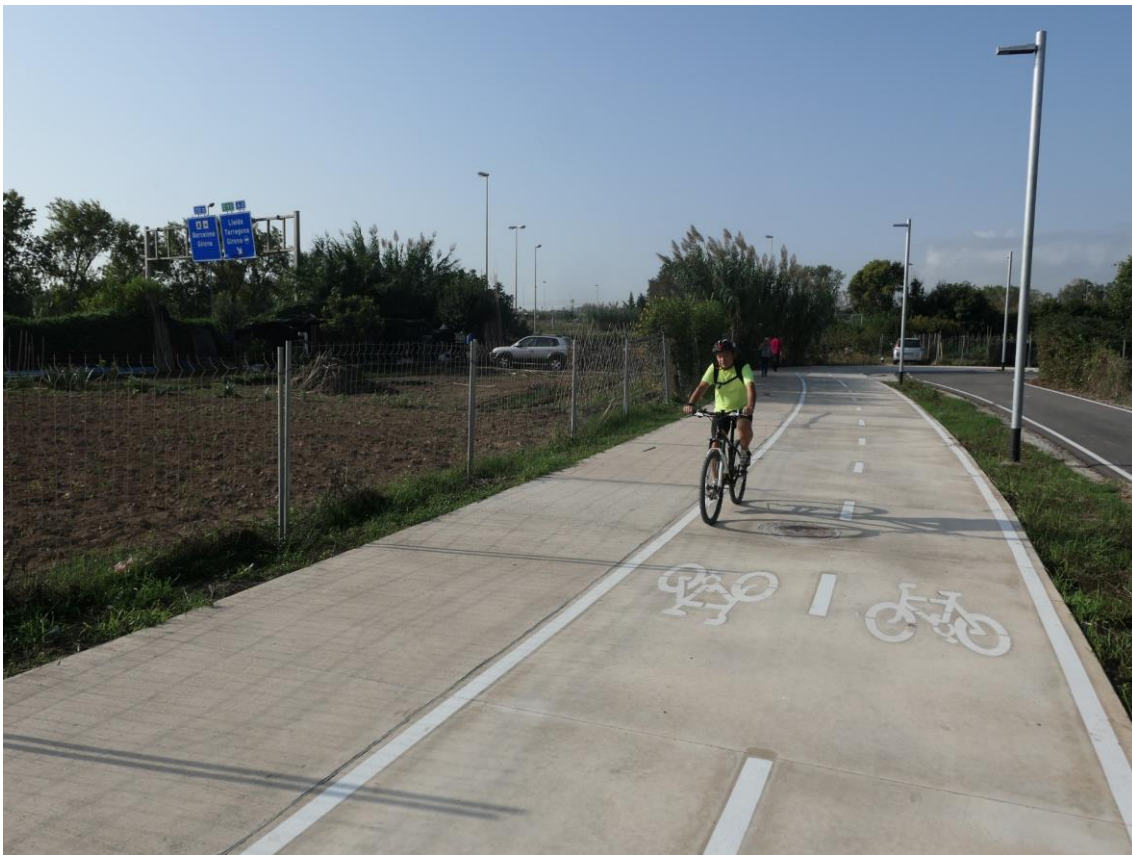
The new metropolitan bikeway Bicivia 7 and sidewalk in the lower Llobregat. C-245 road is to the left © P. Lacroart / L'Institut Paris Region
