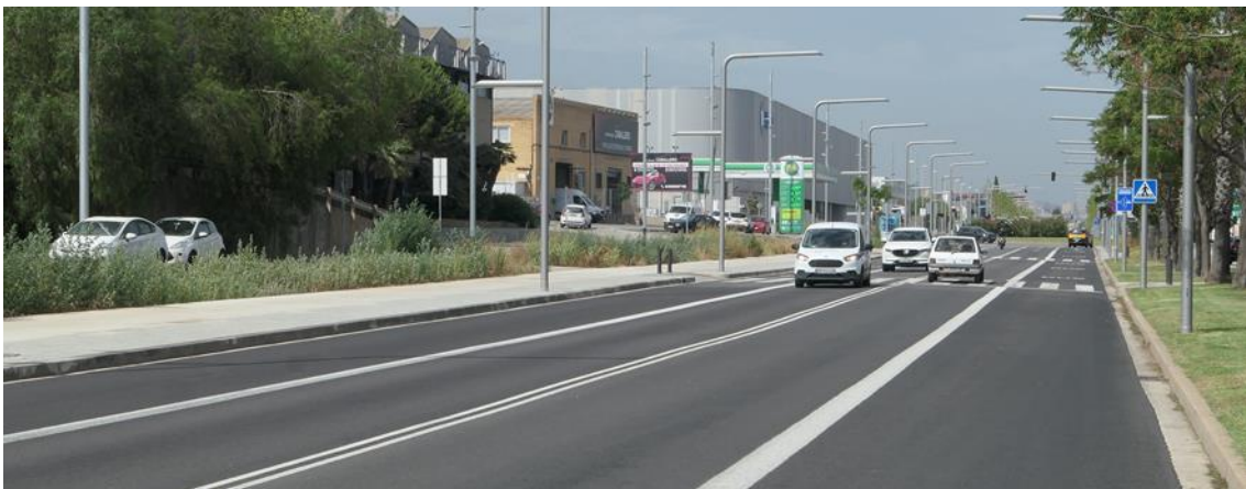
The new C-245 with widened sidewalks, 2+1 bus lanes and 2+1 lanes for general traffic © P. Lecroart / L'Institut Paris Region
