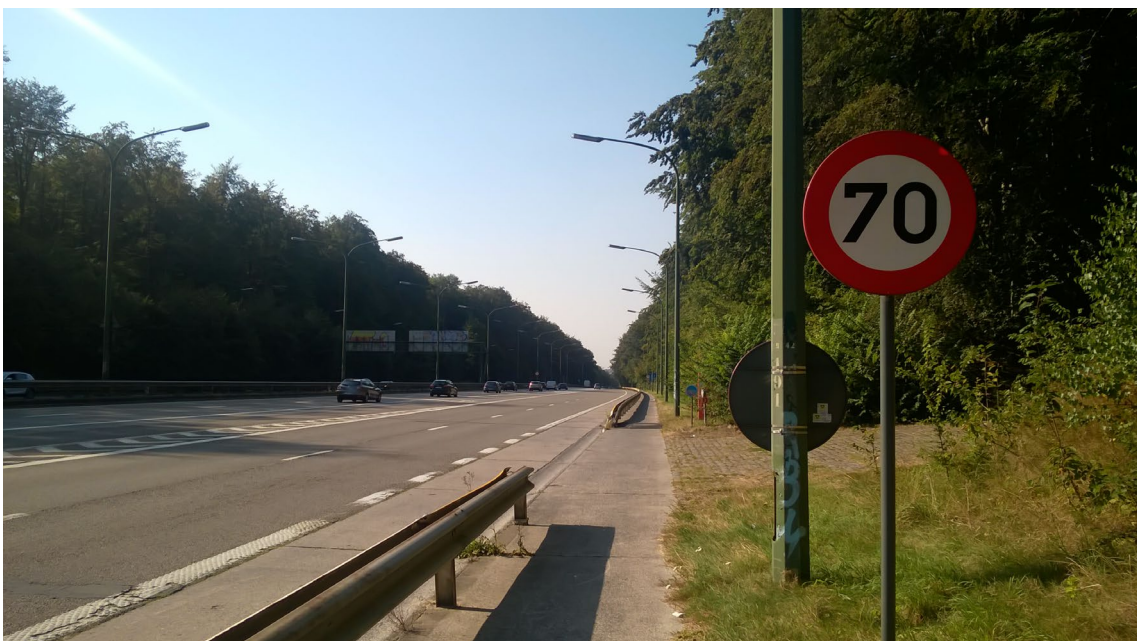
The E411 motorway cuts through the Soignes Forest creating a major environmental scar. Here, the northern roadway going into the city is in the Flemish Region while the southern roadway is in Brussels-Capital Region. Cooperation between the two regions is a challenge for the transformation project.
