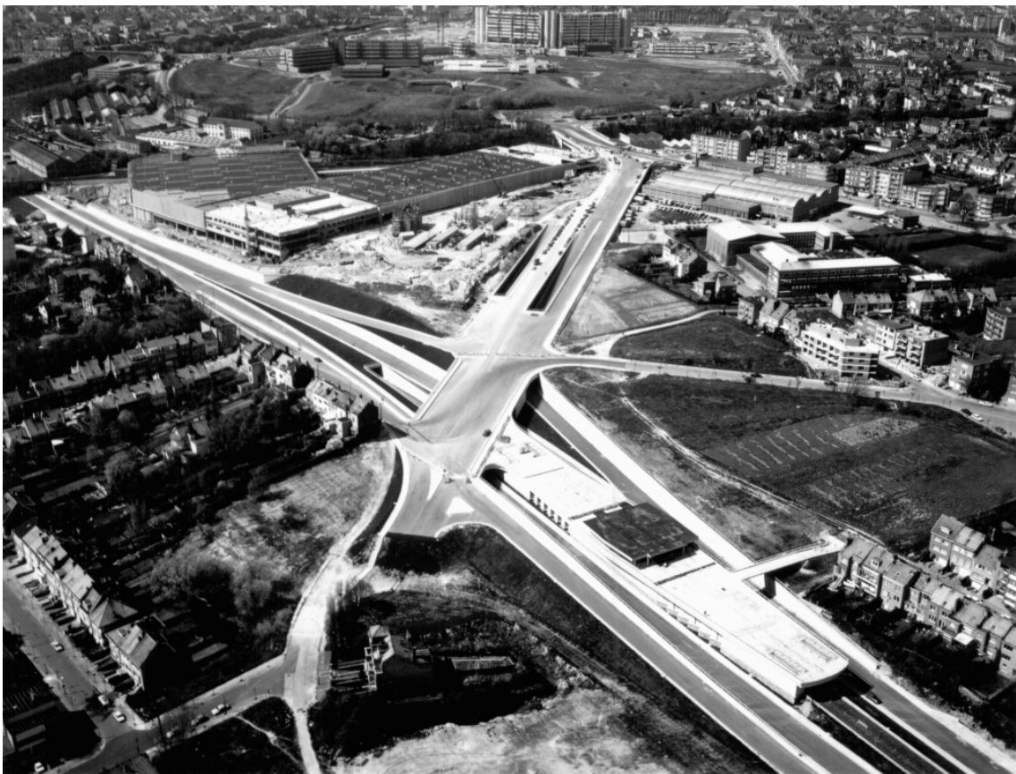
The E411 in construction in the early 1970s brutally cutting across Auderghems' residential neighbourhoods. Above, the Demey-Beaulieu area along the railtracks. Bottom, the Beaulieu metro station built in the median of the highway with STIB Delta area in the background.
