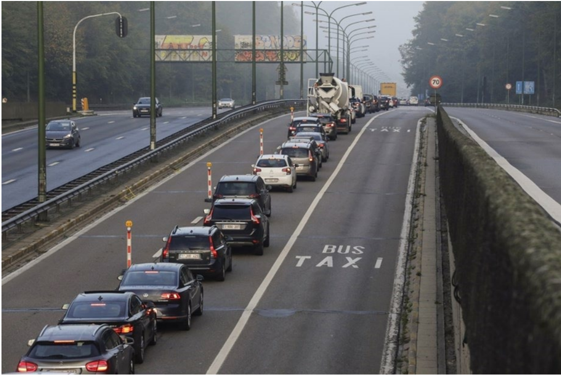
Traffic jam on E411 at carrefour Léonard as it approaches Brussels in 2017 after closure for inspection of the Hermann-Debroux viaduct. © Belga
