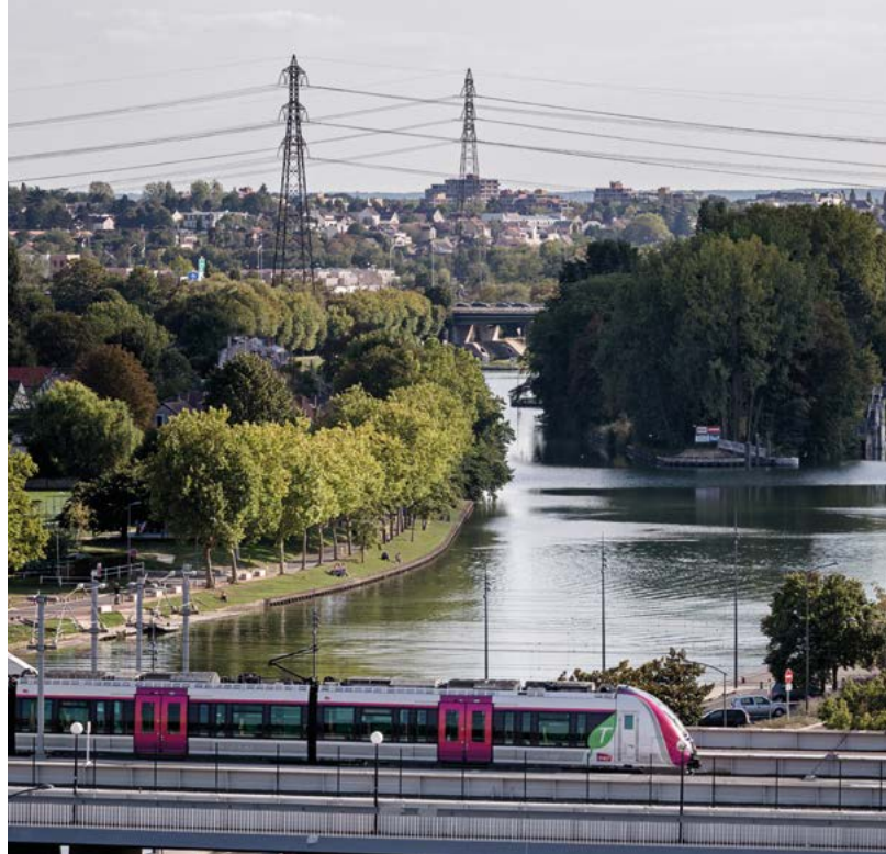
Railway bridge over the Oise © Pierre-Yves Brunaud - L'Institut Paris Region
