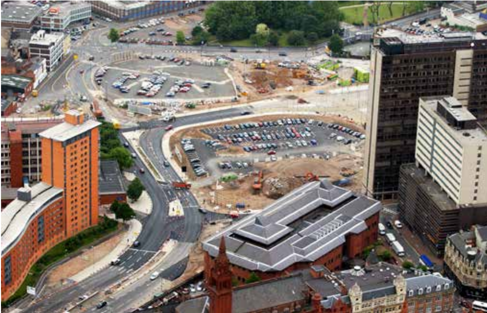
Birmingham: Masshouse Plaza begins to take shape in early 2000s. Copyright: BPM Media
