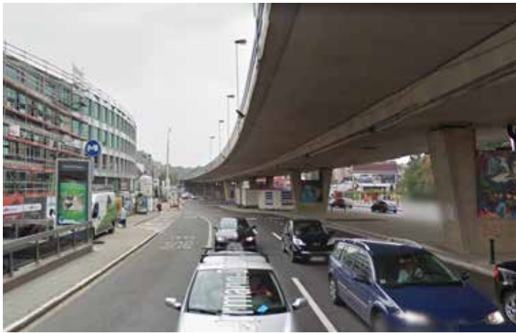
Before: existing street view at Herrmann-Debroux metro
