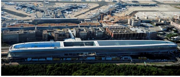
The squaire, a groundscraper located in Francfort Airport City (Hub of Star Alliance), is one of the largest office building in Germany and use by Fraport to attract international companies such as European activities of KPMG.
